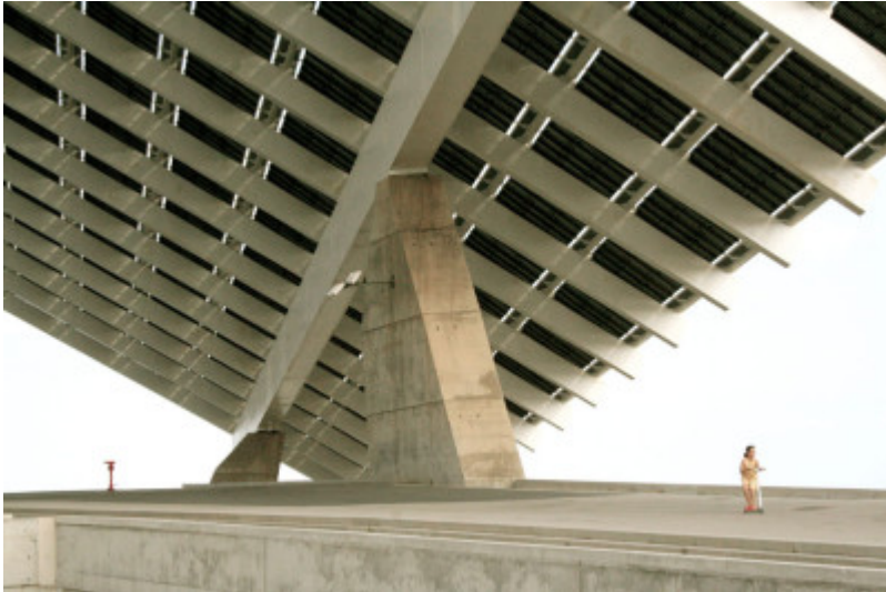
Under Barcelona's solar array at the beach
