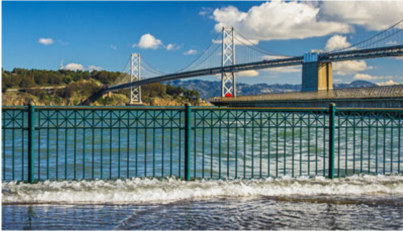
Overtopping Embarcadero, San Francisco, during king tide. Courtesy California Coastal Commission, Photo © Mike Filippoff
