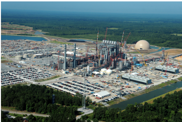
Kemper County Coal Gasification Plant, by XTUV0010
