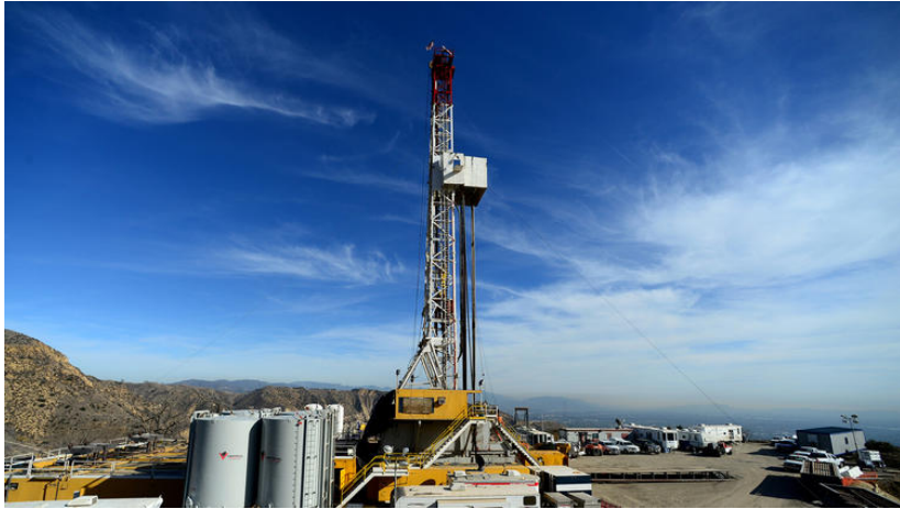
Crews work on a relief well at the Aliso Canyon facility above the Porter Ranch area of Los Angeles in December 2015. (Dean Musgrove / Associated Press)
