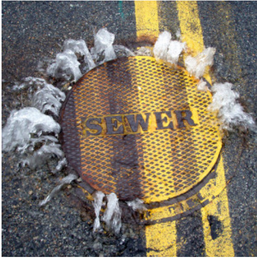
An SSO spills out from beneath a manhole cover. Photo, “Sewer overflowing,” used with permission from Mystic River Watershed Association.
