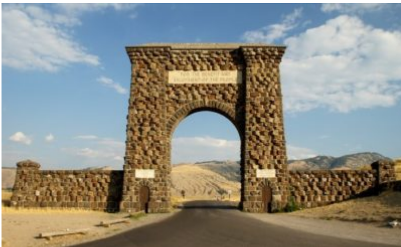
The Roosevelt Arch, marking the northern entrance to Yellowstone National Park.
