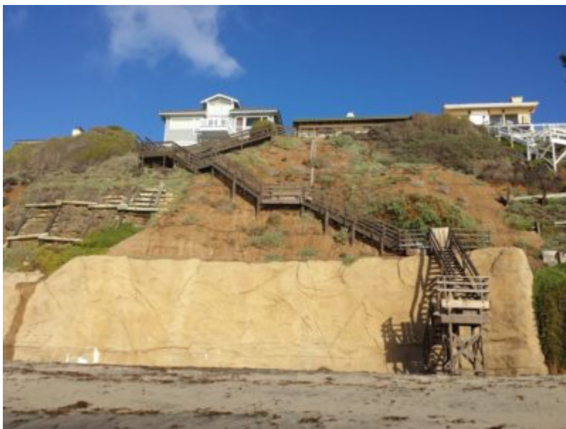
Rebuilt seawall shown in 2012, courtesy of the LA Times
