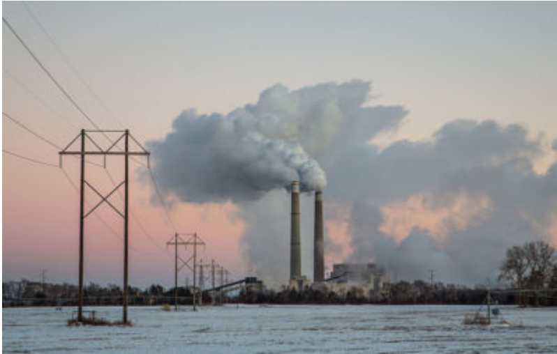
Xcel Energy's Sherburne County (Sherco) Generating Station, a coal-fired power plant, near Becker, Minnesota, Tony Webster. Licensed under the Creative Commons Attribution-Share Alike 2.0 Generic license.
