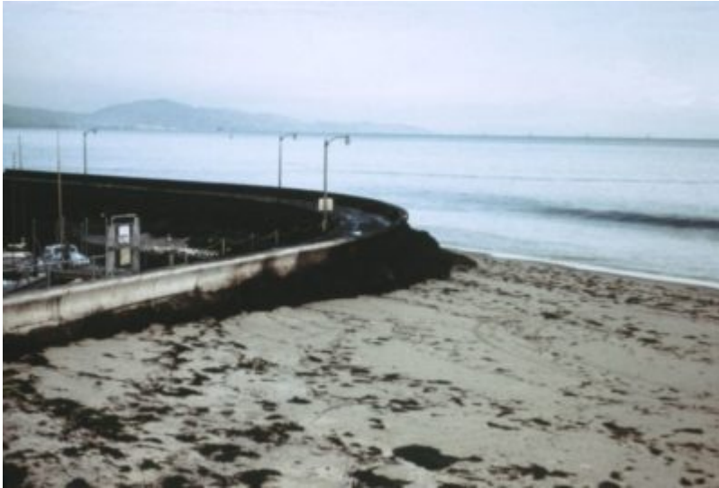
Oil abutting the Santa Barbara Harbor seawall.
