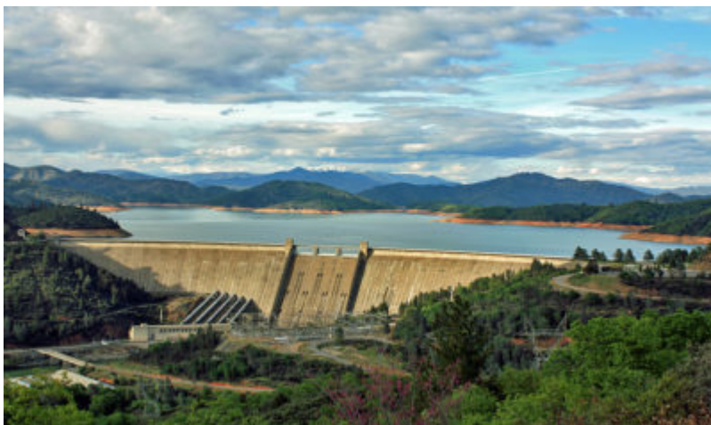
Shasta Dam, Shasta County, CA
