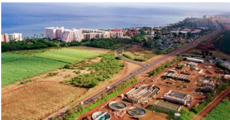
The wastewater treatment facilities at issue in the
