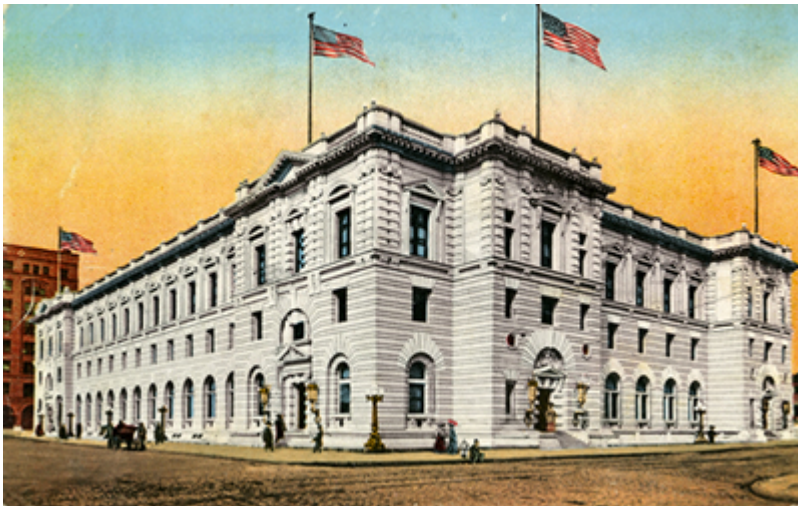
Ninth Circuit Court of Appeals Courthouse, San Francisco, CA
