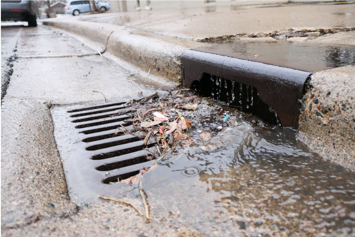
Stormwater runoff flows from a street gutter into a stormdrain in an urban environment. Photo credit: "Polluted Runoff" by Mississippi Watershed Management Organization, from flickr (used under CC BY-NC 2.0)
