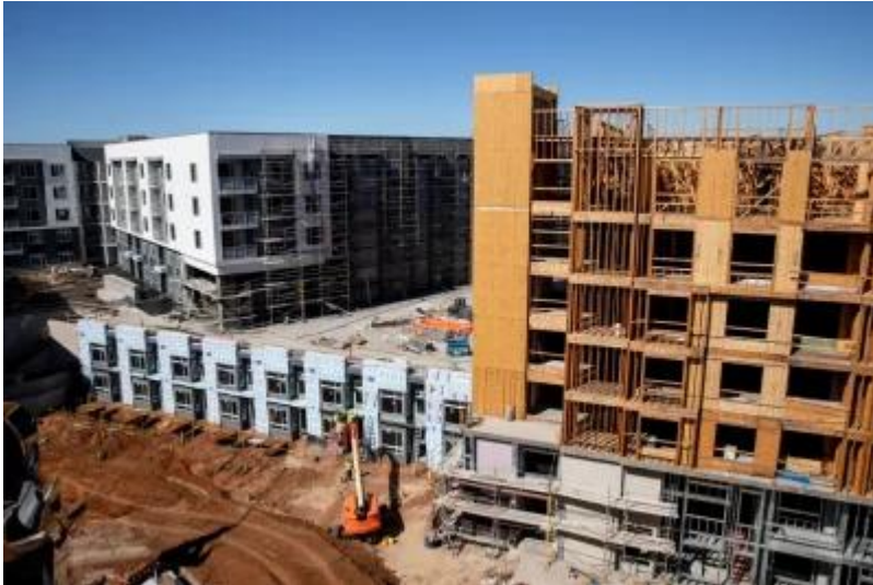
New Apartment Construction in San Diego County (Credit: San Diego Union Tribune)
