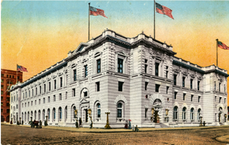
Ninth Circuit Court of Appeals Courthouse, San Francisco, CA (credit: Ninth Circuit Court of Appeals)
