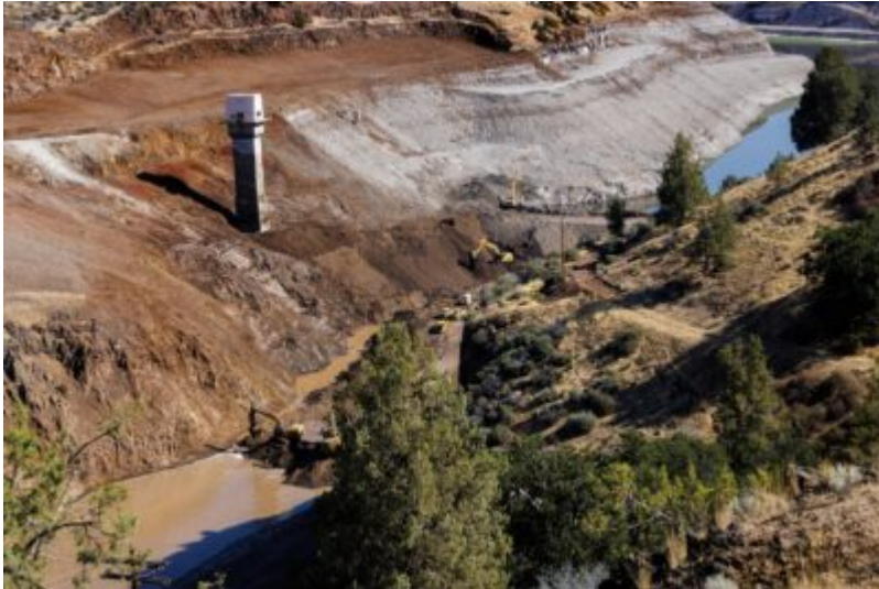
(Klamath River Dam removal project [credit: Los Angeles Times])
