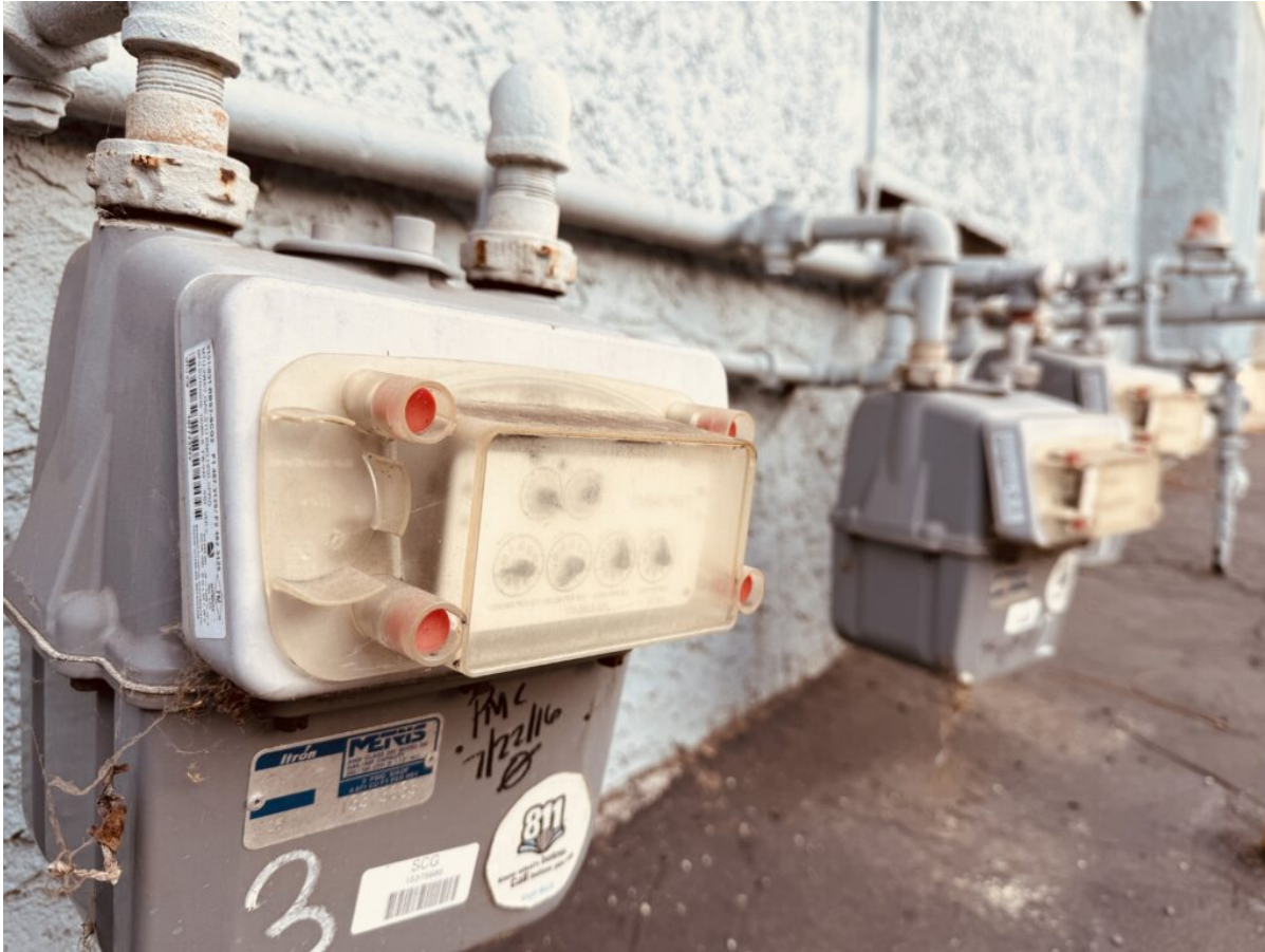
Gas meters for an apartment complex.
