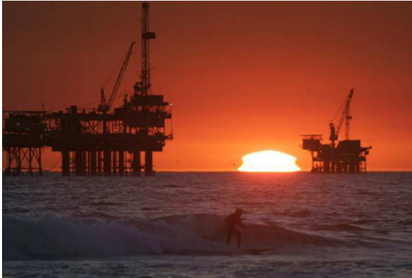
Oil platforms off Huntington Beach (from Greenspace, LA Times)
