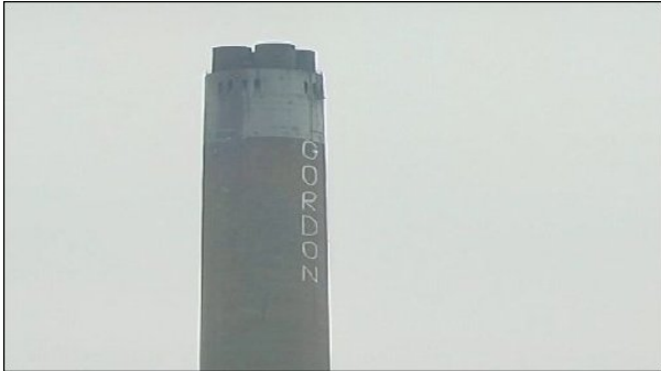
The partially painted tower at the Kingsnorth power station. Photo: BBC News
