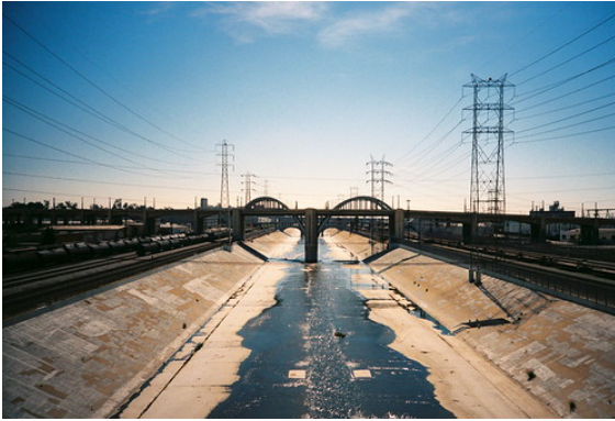
Los Angeles River and 6th street viaduct.
