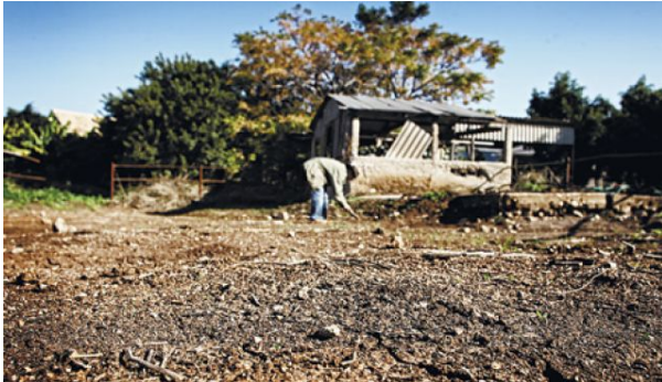
Friable asbestos flying around Nahariya
