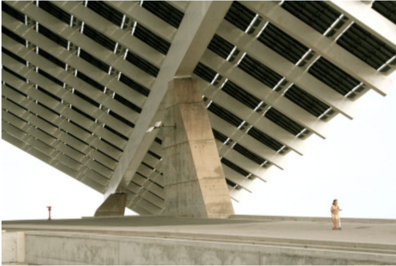
Under Barcelona's solar array at the beach
