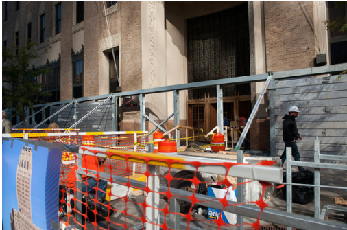
Verizon's New Barrier
