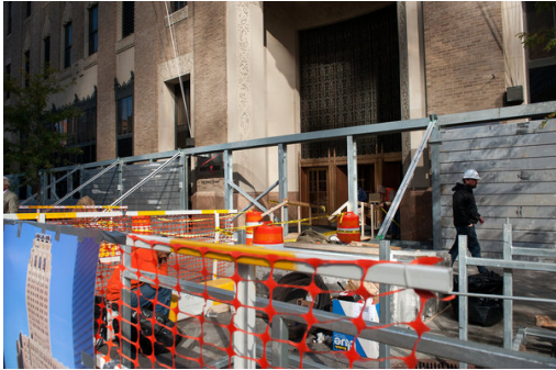
Verizon's New Barrier
