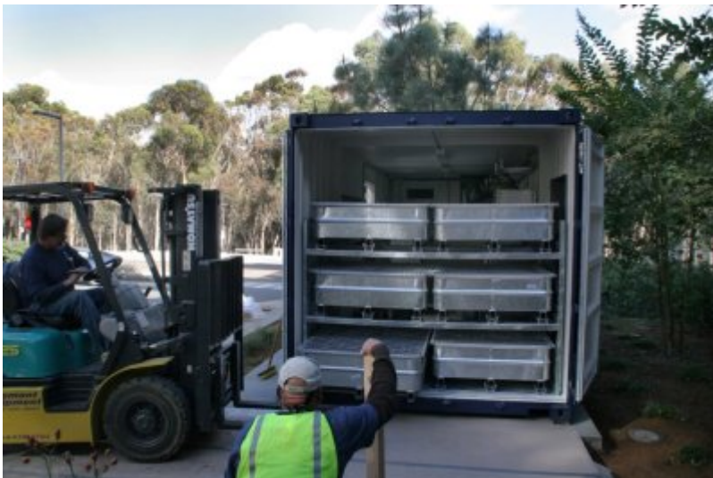
UCSD “second life” EV battery demonstration project. Courtesy of UC Regents/Rhett S. Miller.
