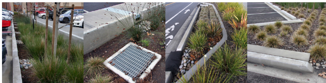
Green stormwater infrastructure includes bioretention systems. (Photos by Nell Green Nylen)
