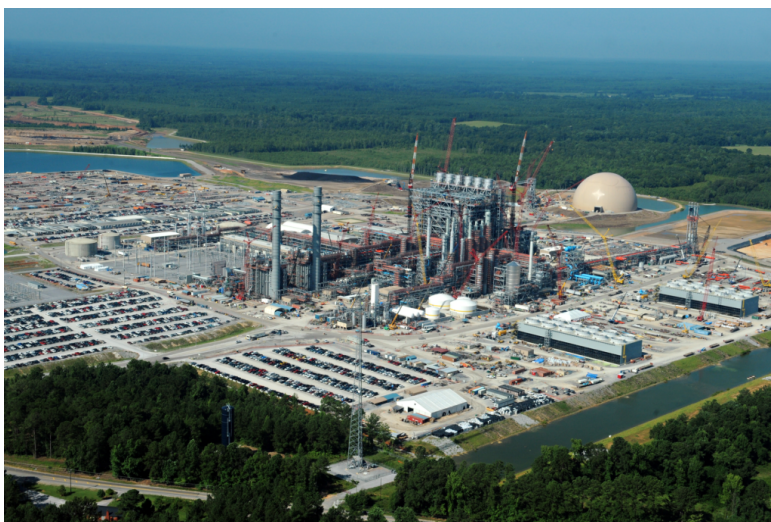
Kemper County Coal Gasification Plant, by XTUV0010
