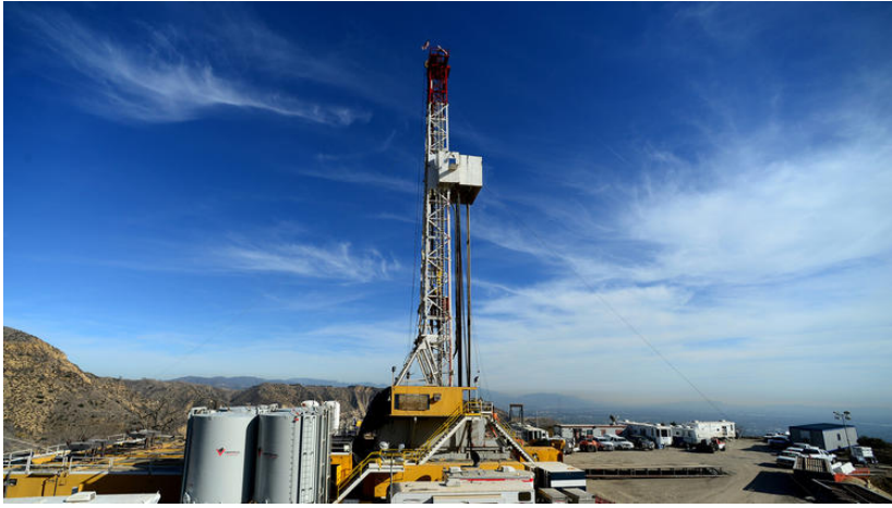
Crews work on a relief well at the Aliso Canyon facility above the Porter Ranch area of Los Angeles in December 2015. (Dean Musgrove / Associated Press)
