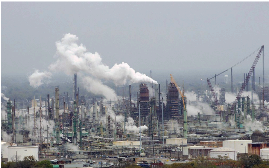
Exxon Mobil refinery in Baton Rouge, Louisiana (WClarke, Wikimedia Commons)
