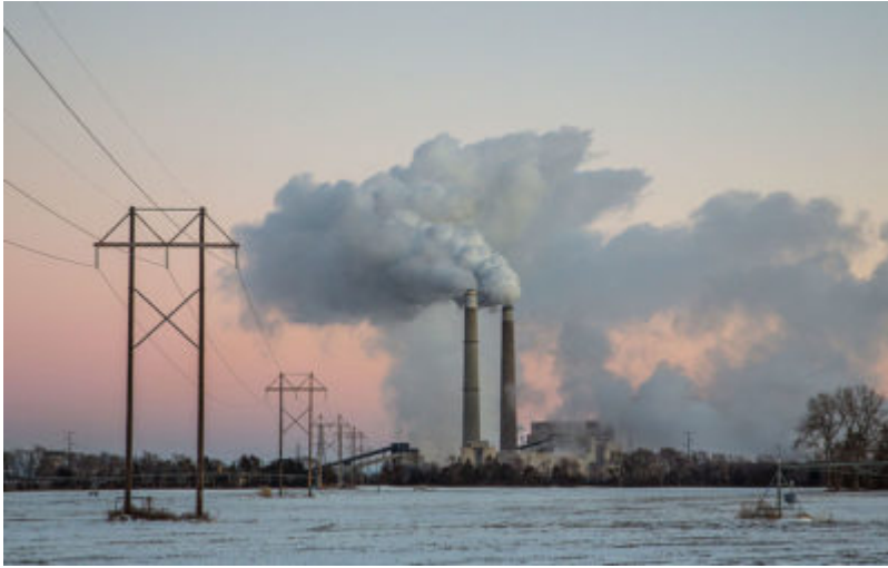
Xcel Energy's Sherburne County (Sherco) Generating Station, a coal-fired power plant, near Becker, Minnesota, Tony Webster. Licensed under the Creative Commons Attribution-Share Alike 2.0 Generic license.
