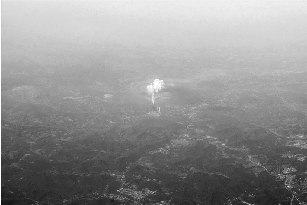
John E. Amos coal-fired power plant in West Virginia, visible from a passing airplane. (Flickr, John Leszczynski)
