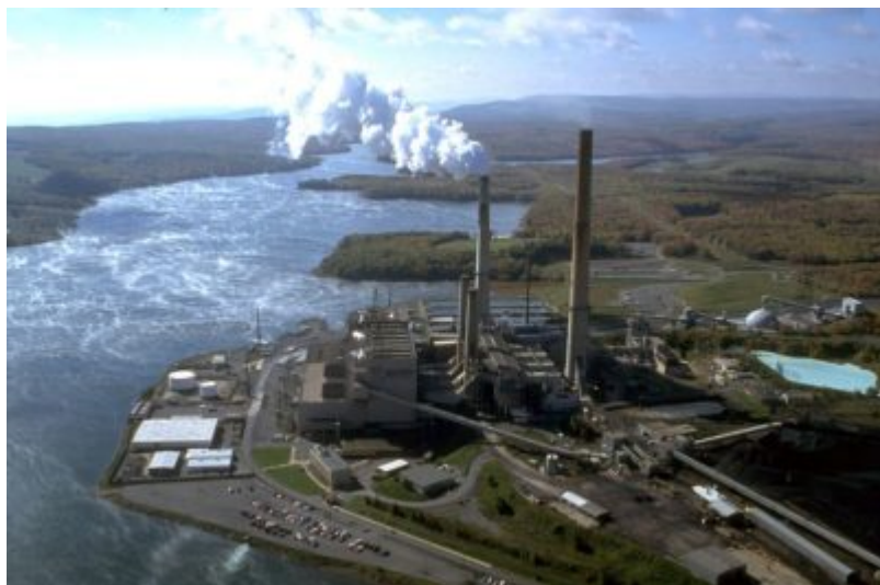
Mt. Storm Power Station, West Virginia (public domain photo)
