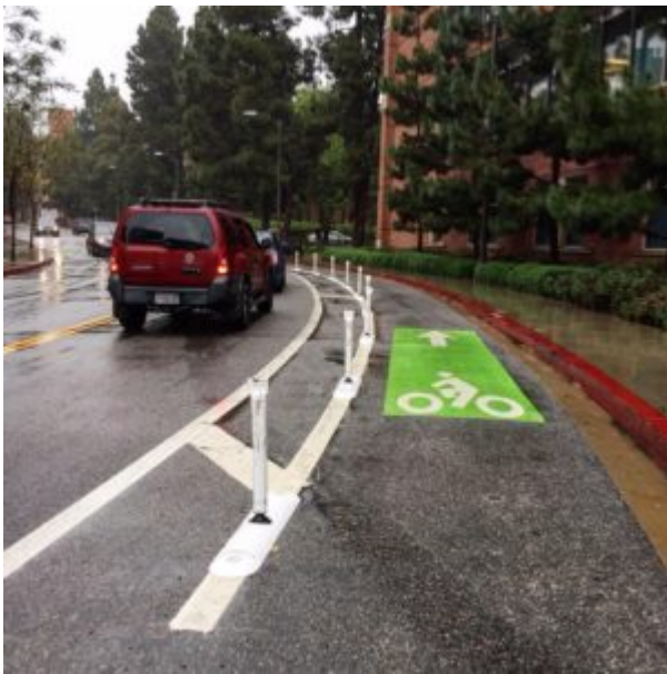
A new, protected bike lane on the UCLA campus. Photo credit: Daniel Melling
