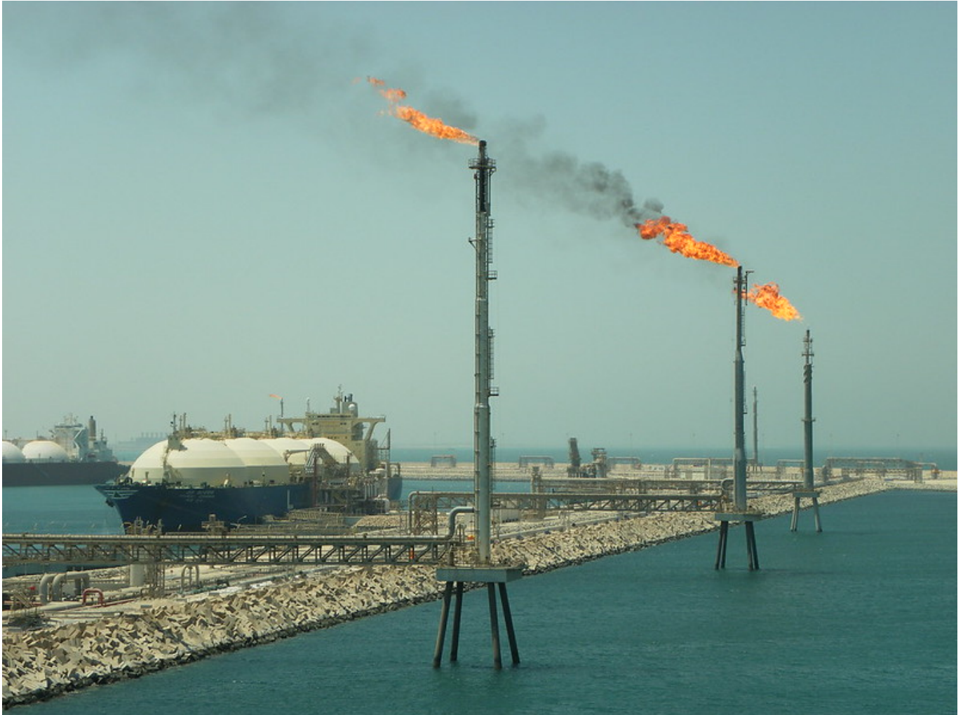
Ras Laffan LNG terminal in Qatar. Photo credit: Matthew Smith, Flickr
