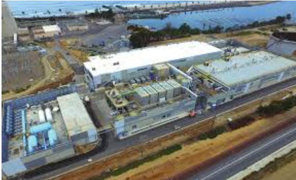
Carlsbad, CA Desalination Plant (credit: sdcwa.org)
