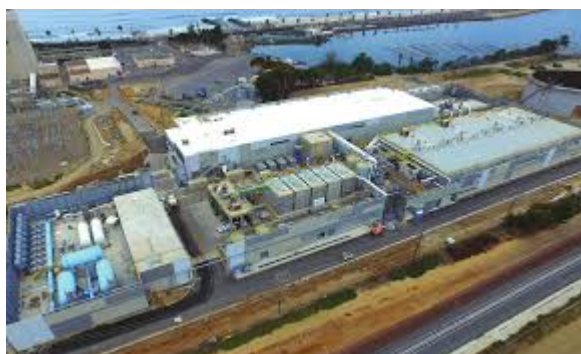
Carlsbad, CA Desalination Plant (credit: sdcwa.org)
