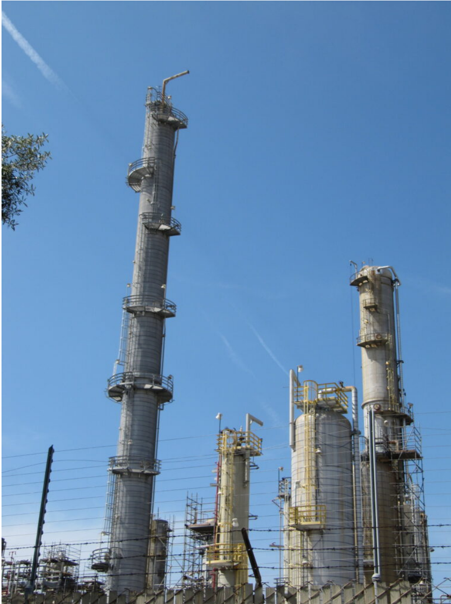
The Torrance Refinery (Flickr, CC BY-NC-ND 2.0)
